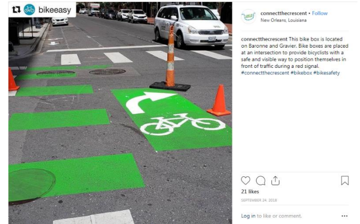
CNO and BikeEasy launched Connect the Crescent, a network of protected bike lanes, in New Orleans Sept 2018 to coincide with the Walk/Bike/Places conference.
